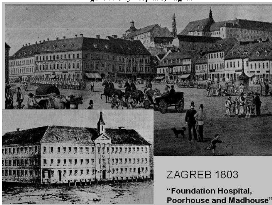
Figure 5. City hospitals, Zagreb
