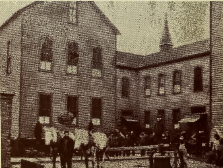
Rear part of former school after it was moved to 50th and Bishop in 1907.
