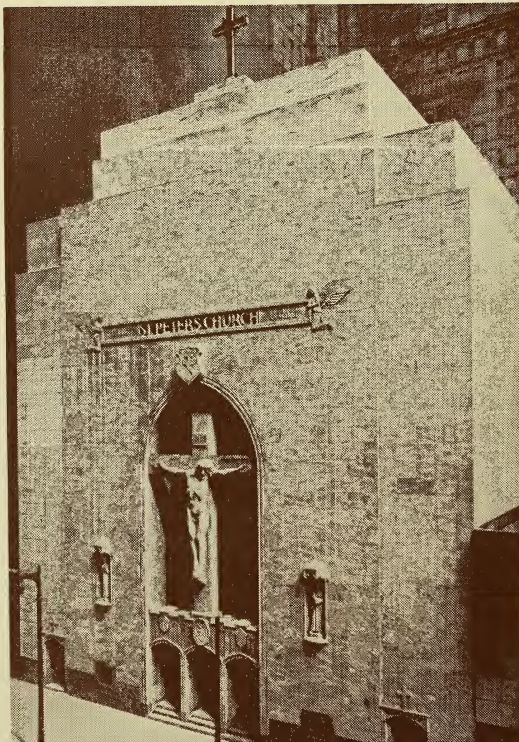
The new St. Peter's in the Loop completed in 1953.
