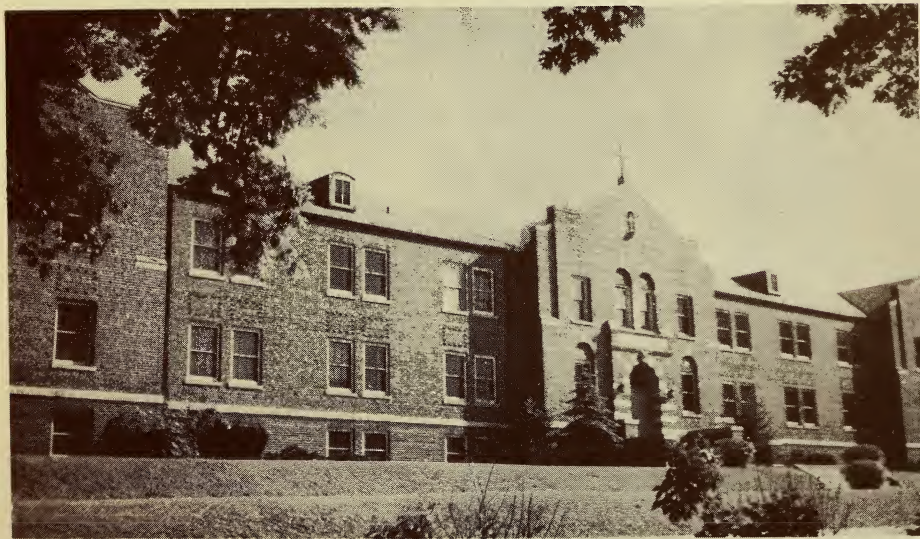
St. Mary's Friary and Seminary at Lemont, Illinois, completed in 1924.
