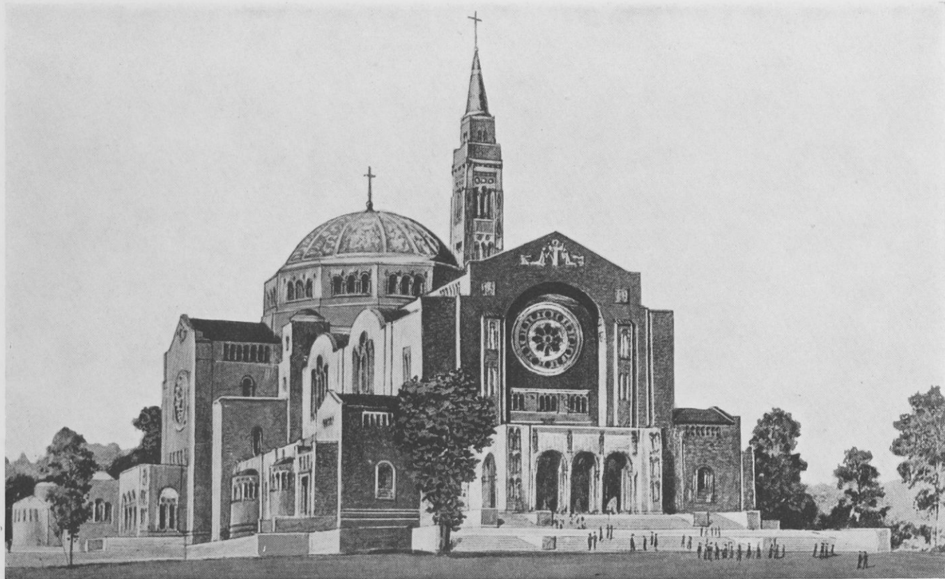
NATIONAL SHRINE OF THE IMMACULATE CONCEPTION (Under Construction)
