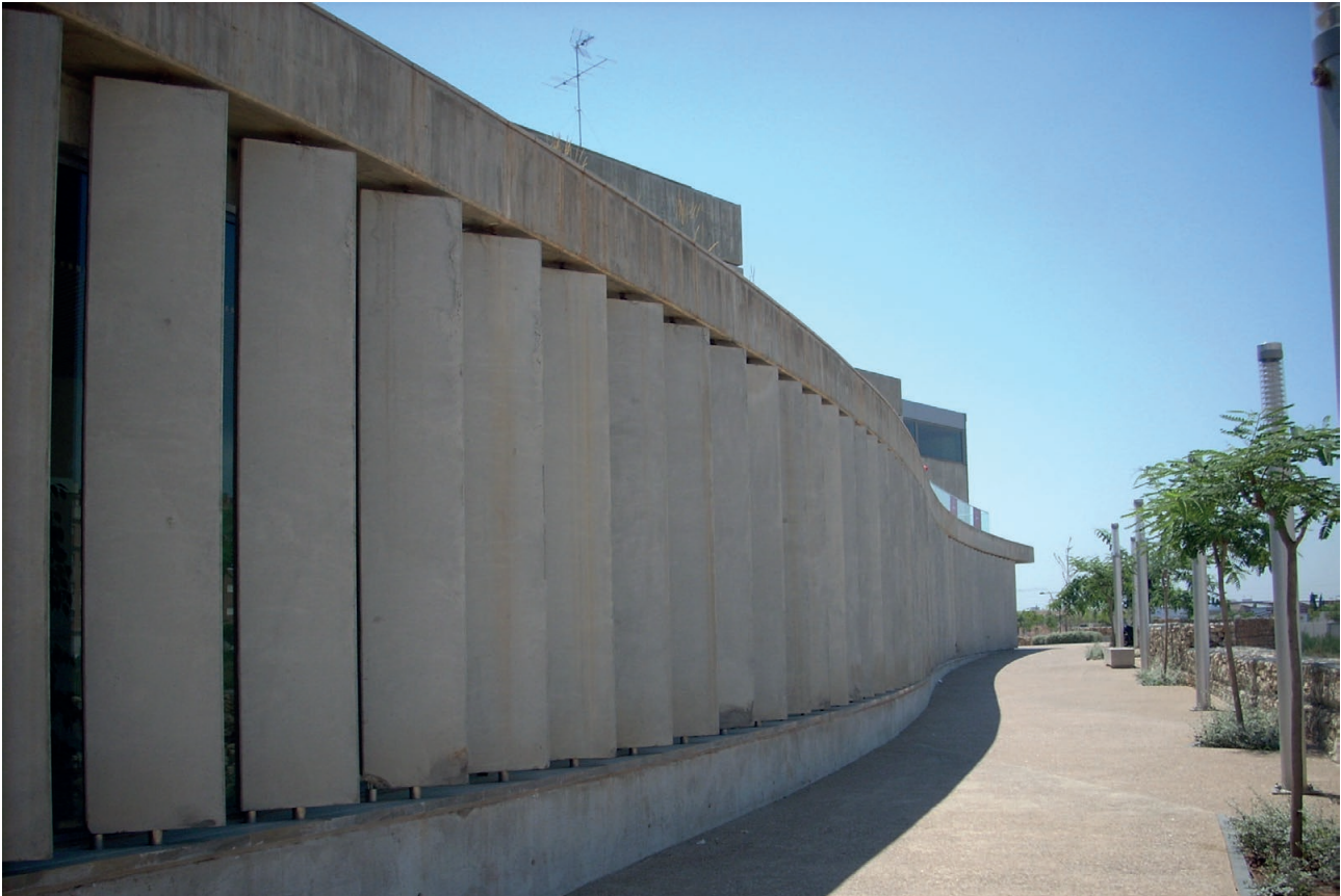
Figure 3 | Swimming Pool and Thermal Centre in Albal, Valencia. Photo: Author's archive.
