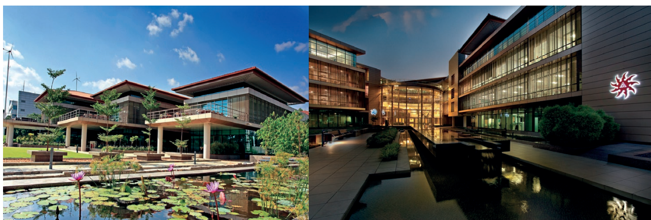
Figure 15 | Sustainable Architecture – Suzlon One Earth Global Corporate Headquarters, India by Christopher Benninger (Christopher Benninger Office, 2019). Prominent Aspects: The objective of sustainable architecture is to minimise the ill-effects of construction on the environment.
