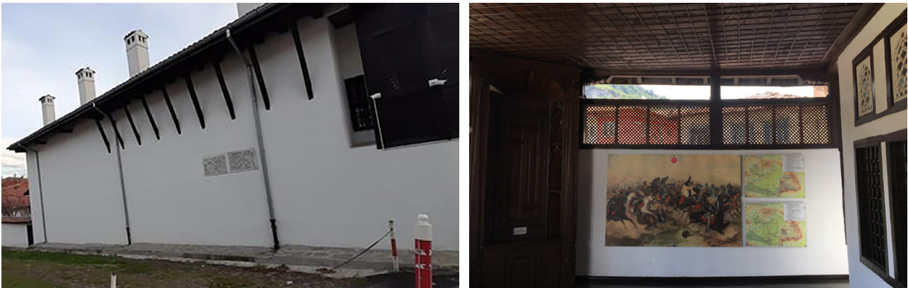
Figure 7 | North (left) façade of the building without any window openings and raised wall of outer sofa (right).
