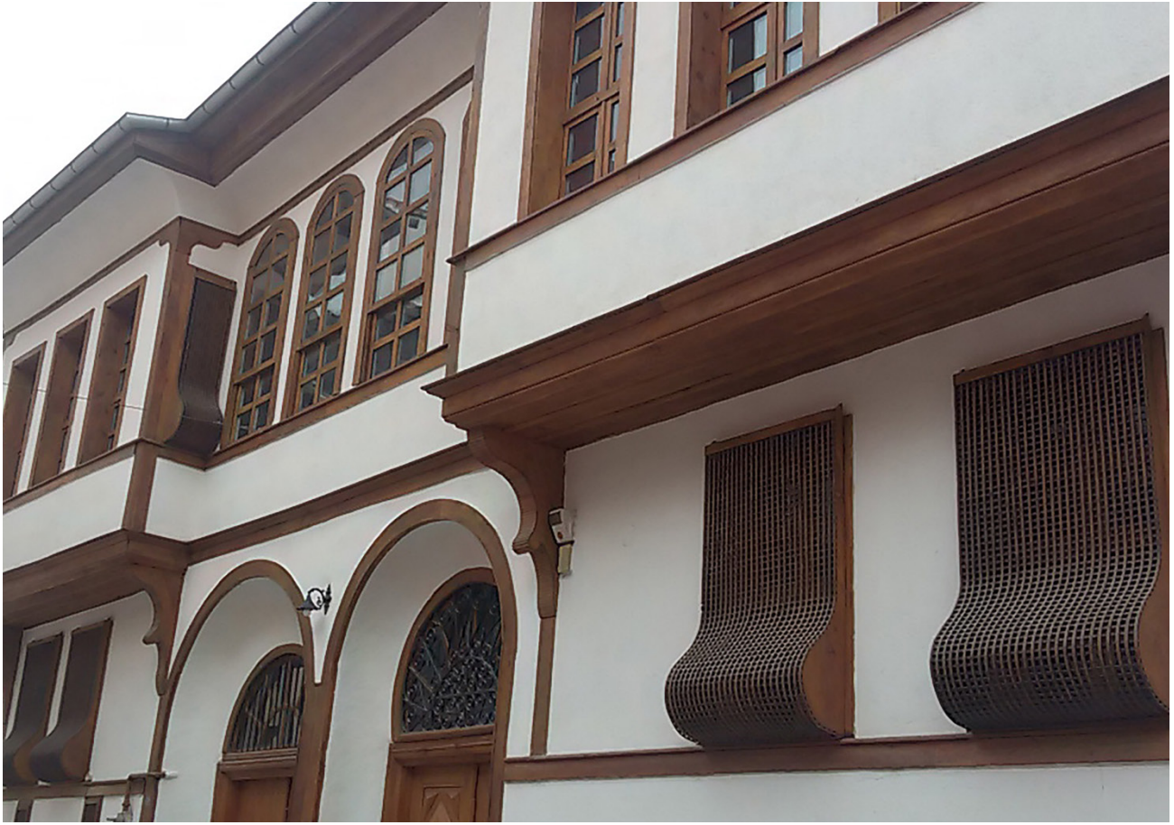
Figure 3 | Wooden shutters for shading for privacy purposes in traditional Kutahya houses.
