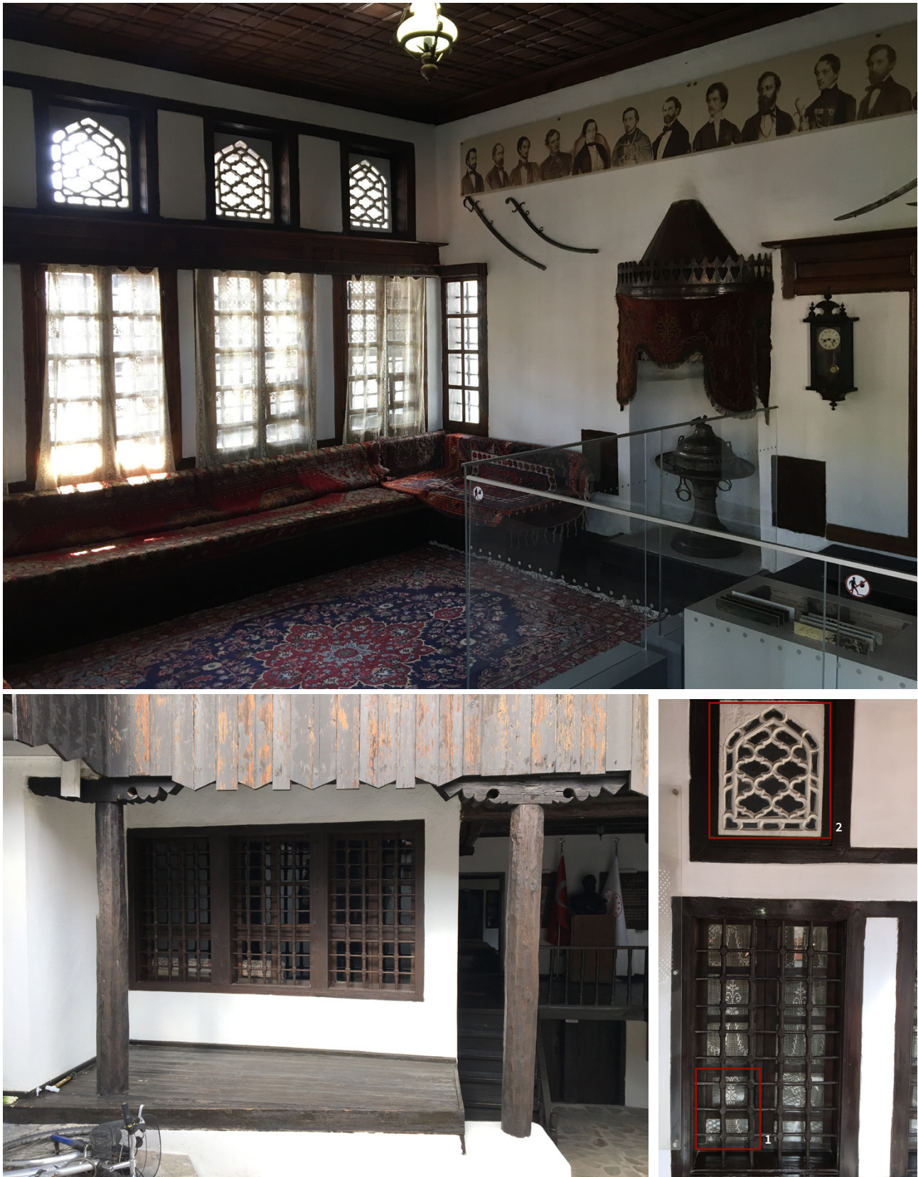
Figure 11 | Exterior and interior views of windows on the winter floor (bottom-left) and summer floor (top and bottom-right) 1: small special opening arrangement used for the ventilation of the room quickly, 2: decorated plaster window at the second row.
