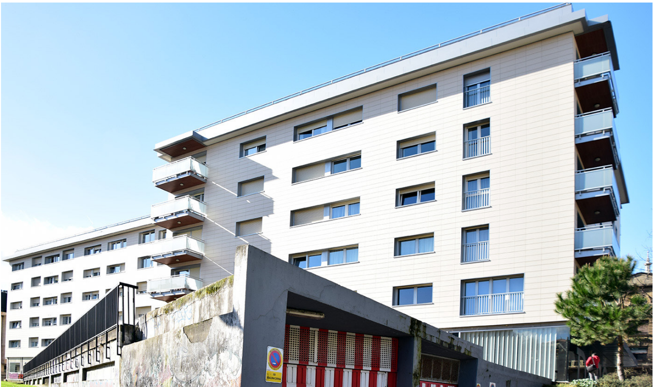
Figure 11 and 12 | Original and current view of the façade of the 60-housing development of the San Sebastián railway cooperative. AHF-A-MSS-Own Archive.
