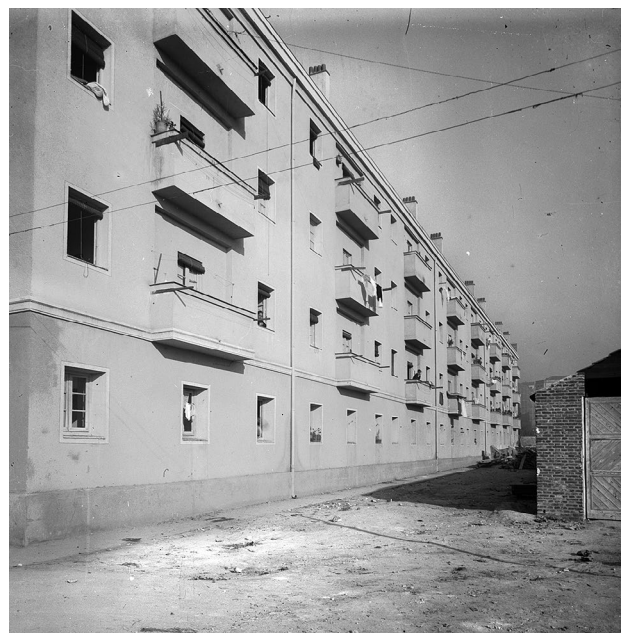
Figure 6 | RENFE, 224 subsidised housing in Madrid-Delicias, 1954. (AHF-ADC-0180).
