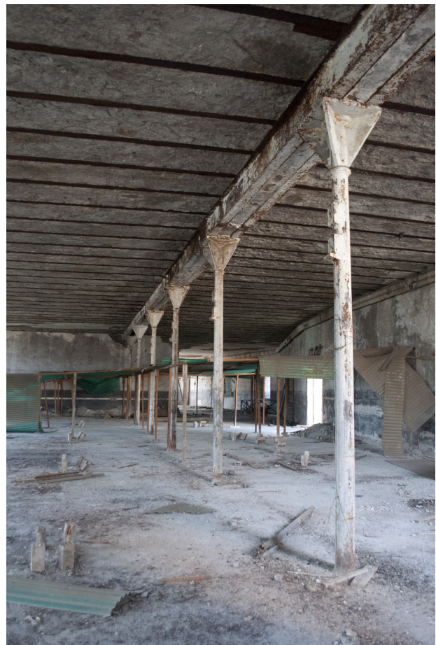
Figure 10. Internal with cast iron columns (by courtesy of Francesco Paolo Longobardi).
