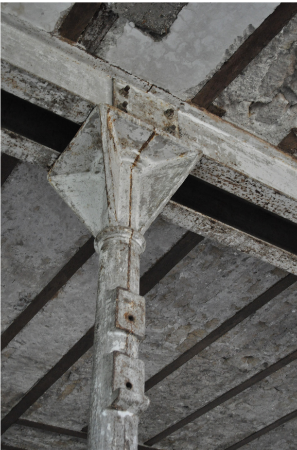
Figure 11. Detail of the cast iron capital (by courtesy of Francesco Paolo Longobardi).
