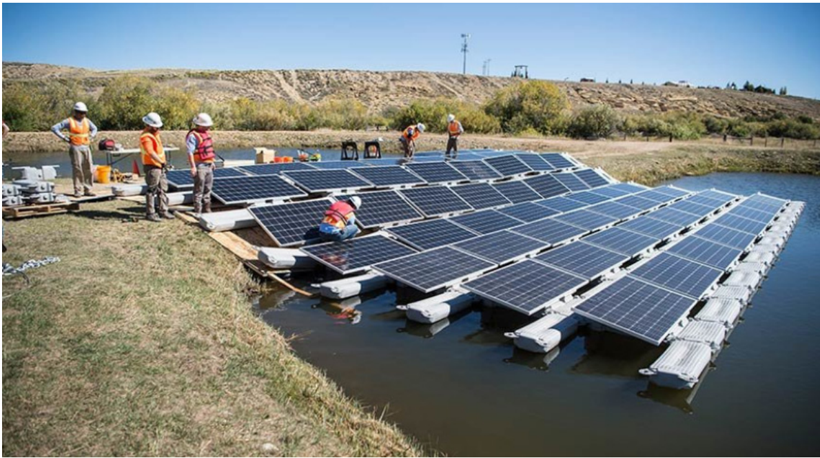
Figure 6. Installation process of the Walden, Colorado Plant. Source: NREL.
