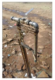
Figure 4: A leaking tap fixed with a forked stick and barbed wire Source: Victor, 2016
