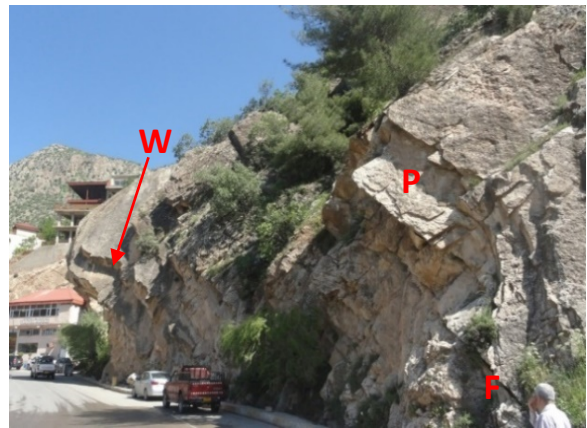
Figure 11. Showing the rockfall (F), and the plane sliding (P), and the wedge sliding (W) at station 3.
