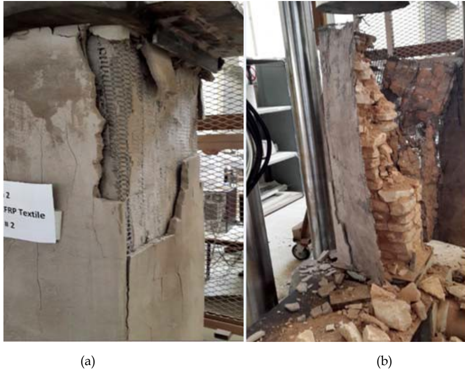
Figure 13. Column CCM2; (a) Outer mortar layer peeled off; (b) TRM jacket opened up at the overlapping and failure of the column.
