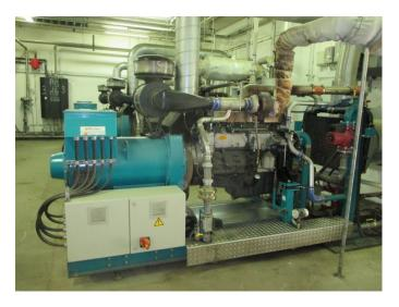
Fig. 2. Demonstration of a co-generation unit in the BS 1 biogas station
