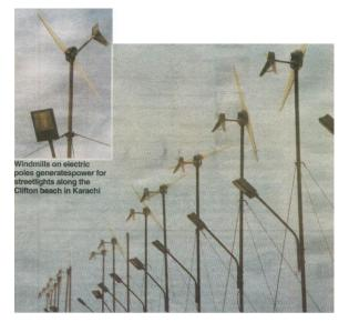
Figure 1: So-called wind farm installed at Karachi Beach and failed after few weeks.
