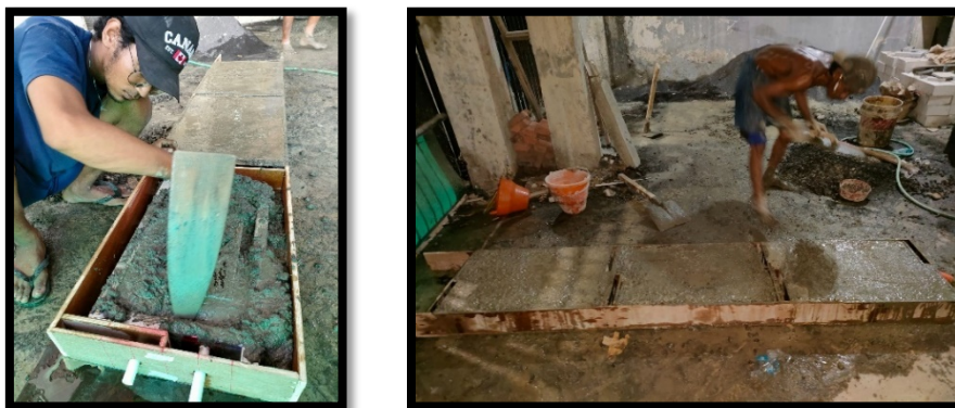
Figure 4. The process of concrete panel fabrication
