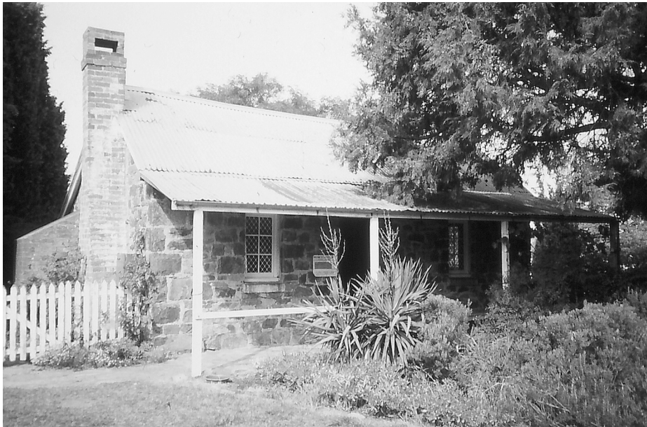
Blundell Cottage 1996. The white picket fence provided by the NCDC restoration of Blundell's Cottage in 1961 has become such a popular fixture that it will be difficult ever to remove. (Photograph Linda Young)
