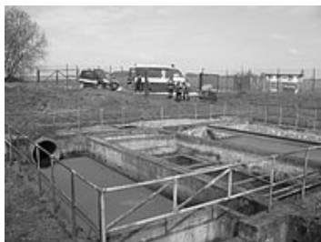
Fig. 1. Lapol D – leaks of oil products.
