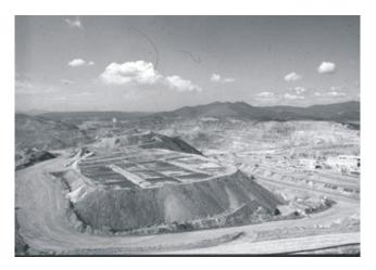
Fig 1 Dump leaching of "run-of-mine" ore at the Kennecott Chino mine, New Mexico.
