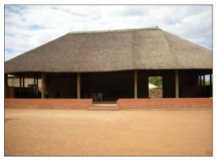
Figure 5: A low-rise masonry wall is used to define the open area with a thatched structure for the elders in a modern-day Kgotla
