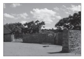
Figure 4: A stone and mortar wall used to form the barrier of the Kgotla (Source: Sebitla, 2018, p. 146)
