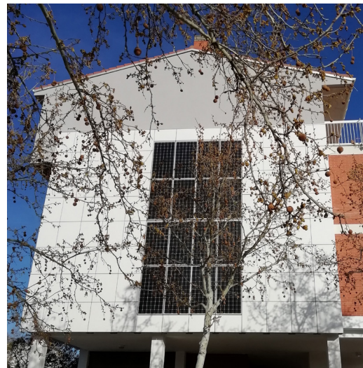
FIG. 12 First demo building installation in Zaragoza (Spain), 2019
