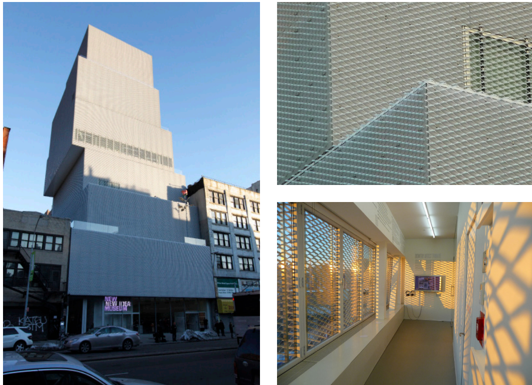
FIG. 2 Example of EM continuous skin. New Museum of Contemporary Art, New York. SANAA architecture office, 2007
