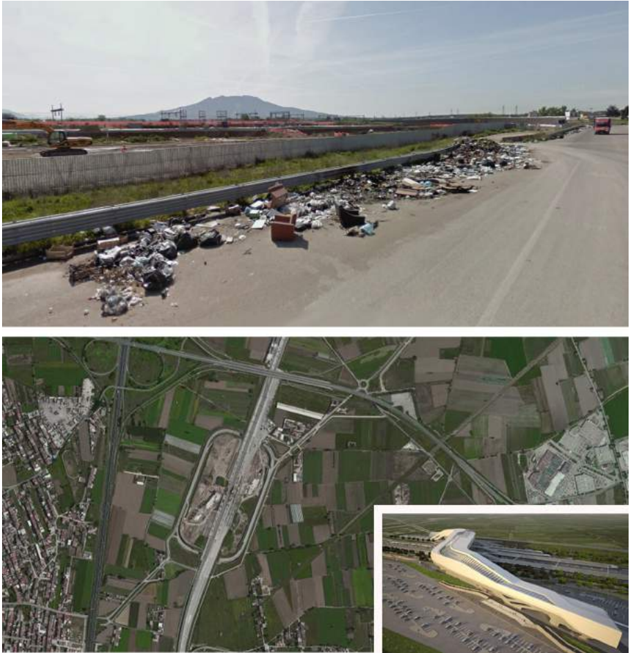
Figure 5 – Work in progress: the new station and the local landscape
