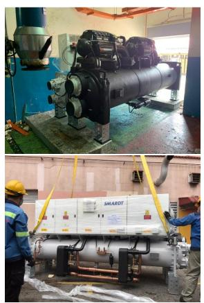
Figure 4. Oil-Free Compressor for Chiller System during Retrofit Program by Energy Performance Contracting with zero initial capital cost
