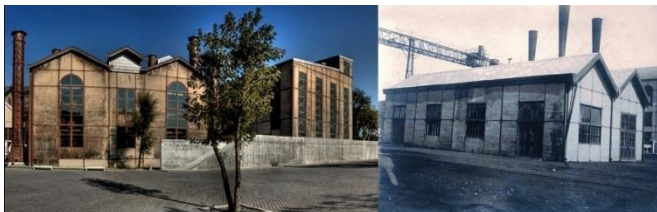
Figure 15. Adaptive reuse in Santralistanbul previous and new building.
