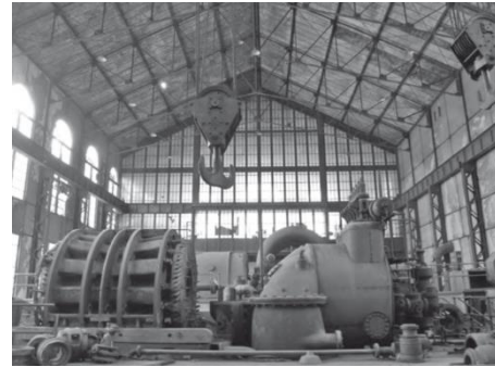
Figure 10. Silahtarača Power Plant, the main machine hall.
