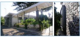
**Figure 21.** Using Iron forks in the right and exposed stone facade in the left (Hera, 2010)
