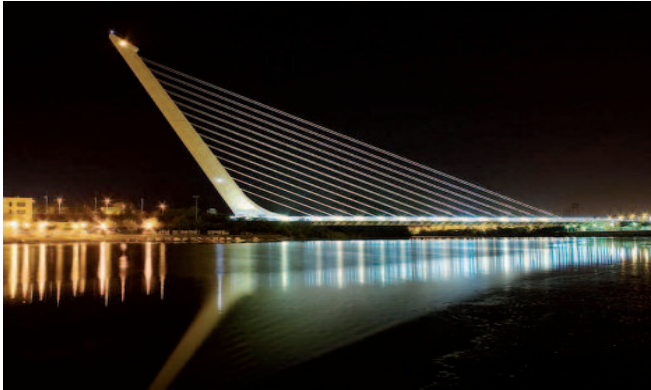
Figure 3. Alamillo Bridge in Seville (Spain).
