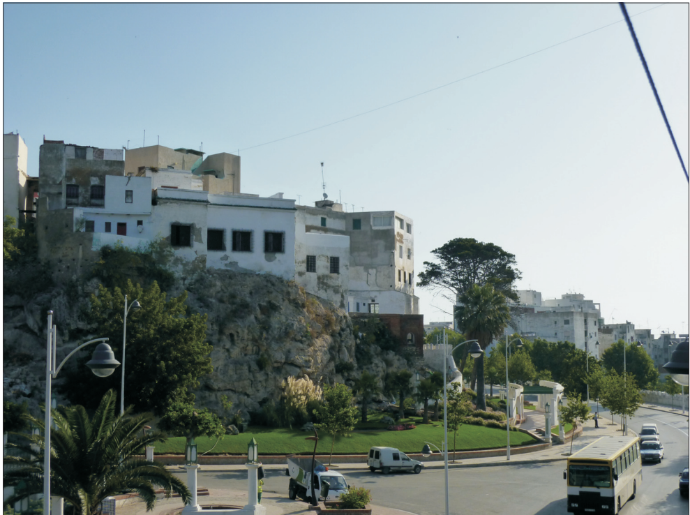
Photo 5. Houses built on travertines in the downtown. Source: Faculty of Sciences, Tétouan, 2013.
