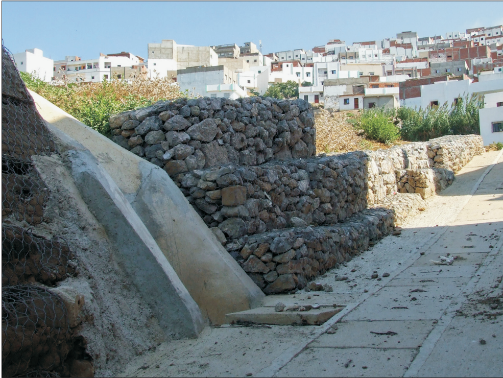
Photo 3. Protective wall between the road and the slope after landscaping (10 x 10 m). (Photo by Prokos, H. 2013)
