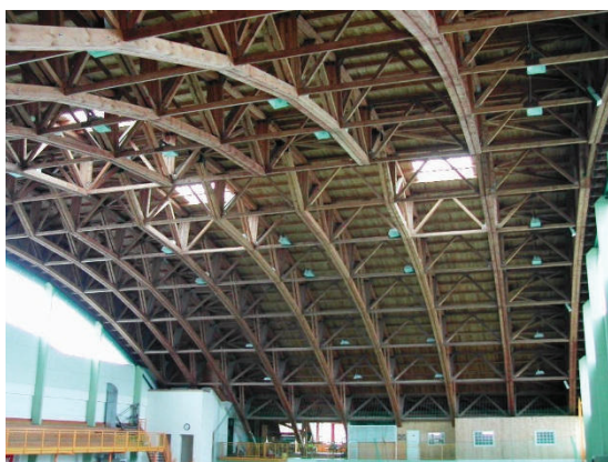
Figure 3: Roof after its completion
