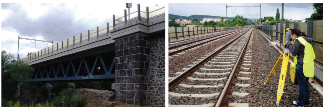
Figure 3: Railway bridge in Klášterec nad Ohří
