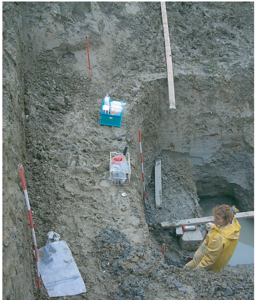
Fig. 6. Large excavation close to the lysimeter at the Avedøre field site. The pit was excavated in steps with vertical and horizontal faces. Profiles were orientated in two directions, perpendicular to one another, so that the fracture characterisation could be expressed in three dimensions. Cored samples from matrix and fracture dominated parts were collected for degradation, sorption and pesticide diffusion studies in the laboratory.
