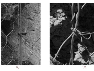
Figure 2: Different connections between the panels: (a) a vertical rope with clips, (b) knots (close view).
