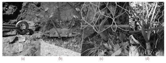
Figure 3: Different anchors types and connection with the ropes and the mesh: (a) a grouted bar with a screwed steel hoop, (b) an injected cable, (c) a grouted bar with a plate, (d) an anchorage plate.
