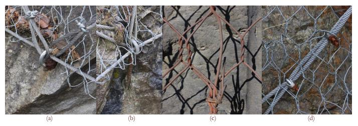
Figure 4: Examples of different damage levels attributed to various components. Different anchors types and connection with the ropes and the mesh: (a) Damage on the plate and/or on the head of the anchors – D1, (b) Unthreading of the anchors – D2, (c) Presence of corrosion and/or removal of the corrosion protections of the mesh – D2, (d) Presence of corroded zones and/or significant damage of the rope – D1.
