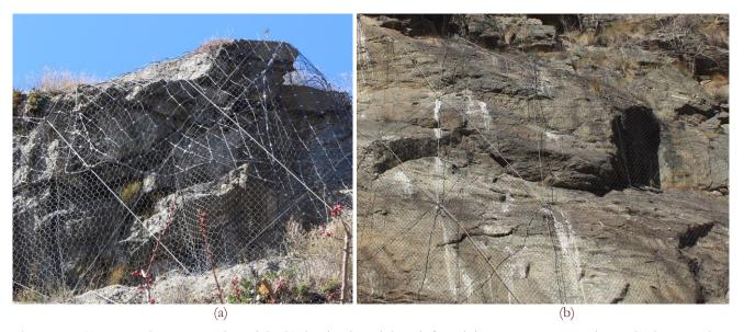
Figure 6: In (a) two mesh types are adopted; in (b) the simple and the reinforced drapery systems are adjacent in the same site.
