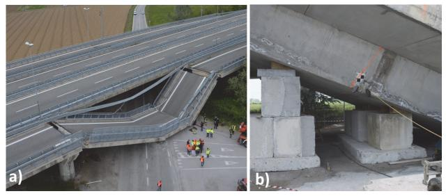
Figure 7: Overview of the collapsed Fossano bridge (a) and structural scheme (b).
