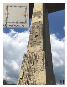
Figure 14: Column details (a); state of decay of the columns (b).
