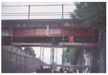
Figure 19: Steel resurfacing for I-beams of an overpass [Copyright: RELUIS].
