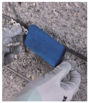
Figure 16: galvanic protection: sacrificial anode [Copyright: Mapei].
