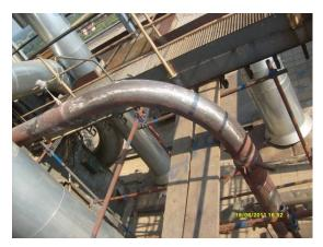
Figure 1: Part of the steam line during NDT.
