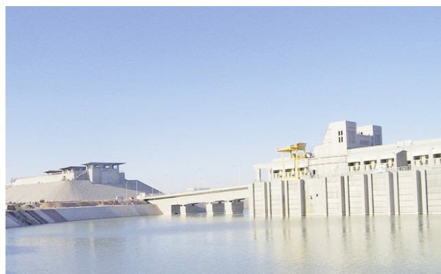
Fig. 1. Toshka Pumping Station
