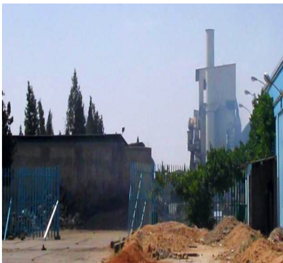
Fig. 5. Chimney of the NCEP complex - lead refining unit.
