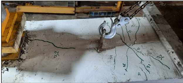
Fig. 11. Crack pattern of specimen S-RL1.5.
