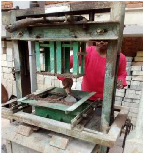
Fig. 2. Use of block making machine for CSEB production.
