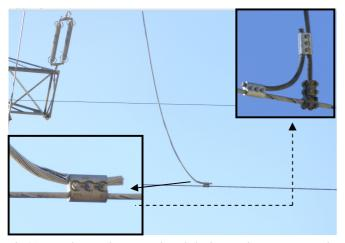
Fig. 21. Broken conductor strands and the improved arrangement at the junction outside the Agia Varvara Substation (the station was constructed as a connection point of a wind farm, an obvious hint that the location is subjected to strong and frequent winds).
