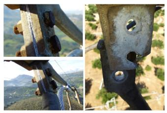
Fig. 17. Views of a severe hot spot.
