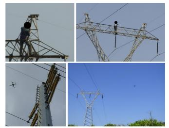
Fig. 12. Climbing and drone inspection. Up: Climbing inspections. Down: drone inspections. Note that a no-zoom drone has to approach to a very close distance (left image) but a suitably equiped drone can perform inspections from a safe distance (right image).
