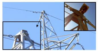
Fig. 9. An overhead shield wire arrangement on a double circuit suspension tower using a yoke plate and dead-end tension clamps to replace the initial suspension clamp, making the arrangement effectively similar to that of a tension tower. Down and left image: a zoom-in of the arrangement. Up and right image: A similar approach on a single circuit suspension tower proved problematic.
