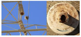
Fig. 6. A jumper part of a tension tower suspended by two coated glass strings (to avoid wind lift-offs). The last insulator of the right string was found unbuckled during inspection. As shown in the right picture, the insulator's cap was found misfigured.
