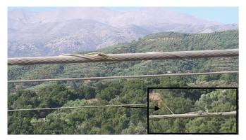
Fig. 20. Broken conductor strands due to vandalism.
