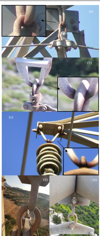
Fig. 13. Inspection photos. (a) and (b): drone photos, (c): photos taken from the ground, using a 60x zoom camera. (d) and (e): climbing inspection views. Pictures within pictures in (a)-(c) are zoomed in details of the larger respective pictures.Notice that even when the viewing angle from the ground allows to spot an issue, the secerity of the issue can not be safely assessed.
