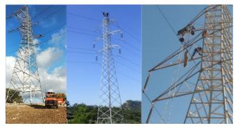
Fig. 10. Maintenance works on double circuit towers with only one of the circuits turned off. Extra care and consideration should be given to the direction of the wind as ropes and pulleys are used to lift tools and equipment to the maintenance spot.
