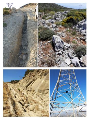
Fig. 14. Maintenance works on the ground: an exposed ground conductor, impassable roads and a hanging angle in a tower's body (noted with an arrow).
