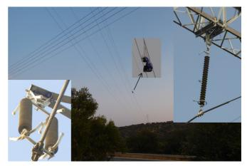
Fig. 11. Views of ground inspections, taken with an 60x optical zoom camera. Left image: A transient arc caused by a bird carrying a string. The arc traces are visible on the arcing horn of the right insulator along with a piece of string. Middle image: a potentially dangerous object on a conductor midway of the span, as seen from near one of the towers (natural and zoomed in view). Right image: a nest right above of an insulator.
