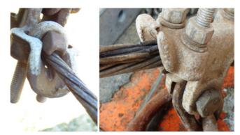
Fig. 8. Overhead ground wire issues: a damaged suspension clamp (left) and broken strands (right)
