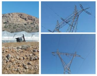
Fig. 5. A car tipped-over by the wind near Atherinolakos (left). Wind liftoff of conductors and/or jumper parts on lines not equipped with additional weights and/or ceramic insulators at jumper parts (right).
