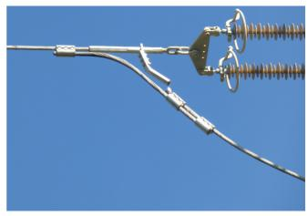
Fig. 18. An additional jumper saving the day.
