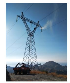
Fig. 4. Dead washing of the Moires-Ierapetra line. The water is carried with trucks and pumped-up to the lineman that performs the washing. The line is to be refurbished and the new footings and base are visible.
