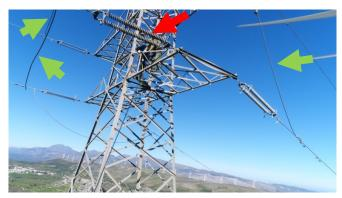
Fig. 5. A direct view of the flashed under insulator (red arrow). Some conductor parts used for phase transposition are also visible (green arrows).
