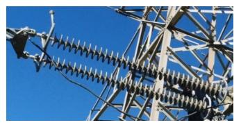
Fig. 8. Even from a small distance, the damage is not visible due to the sheds overshadowing the seath
