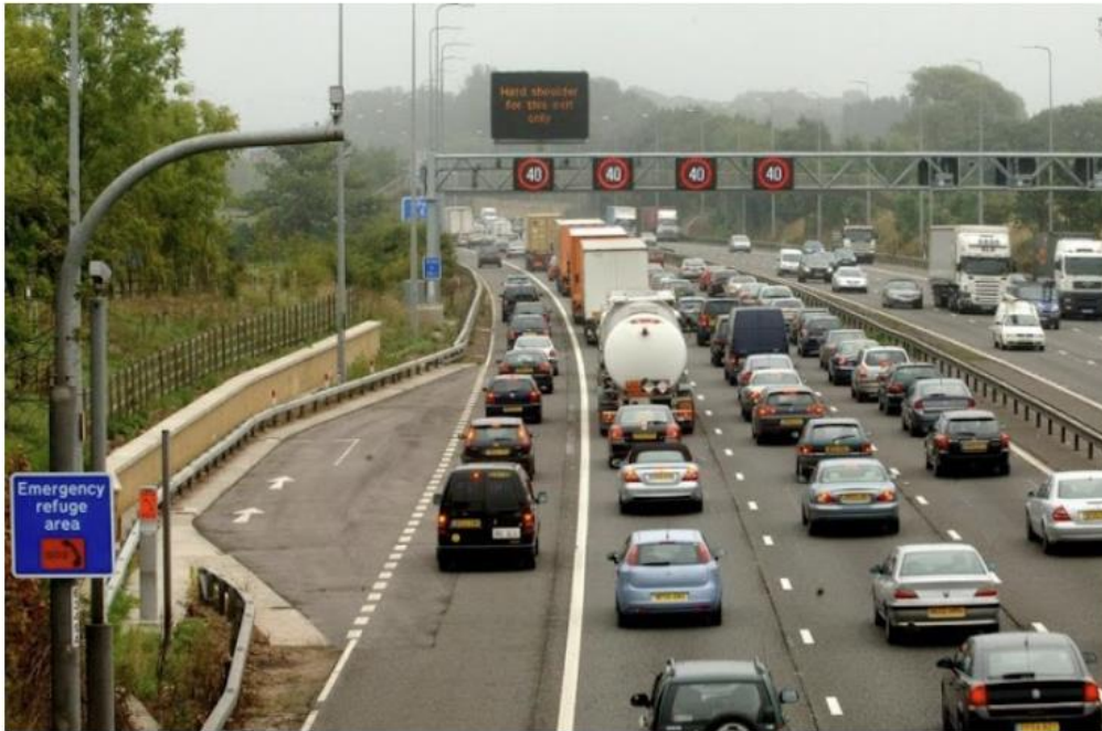
Dynamic smart motorway (revtothelimit, 2021)
