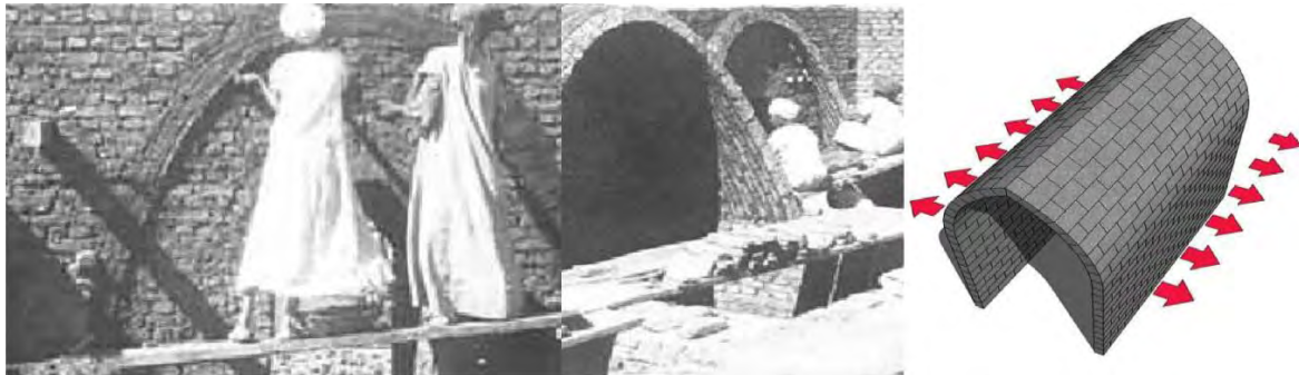
Figure 6. Depicts the roofing methods using the vaults
