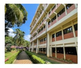
north side where classrooms are located. The glazing materials used is 6mm clear glass with windows size with the area of 1.38m<sup>2</sup> and 2.07m<sup>2</sup> for each opening. The investigation is conducted for floors two to five where classrooms are located along the corridors. This study separates the classroom areas between the north and south facing parts of the building to understand the different illuminances of each area (**Fig. 3**).
