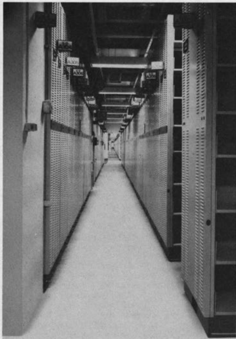
The world's largest installation of movable compact shelving is in the world's most famous library, in Washington, D.C. RHC-Spacemaster manufactured and installed the entire system, including unique microprocessor controlled operating and safety systems.
