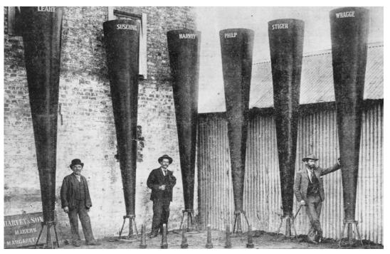
Figure 2 - Battery of Stiger Vortex rain-making guns at Charleville, Australia 1902
