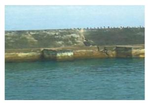
**Figure 2.** Cracking on breakwater concrete wall after an earthquake on January 21<sup>st</sup>, 2012.
