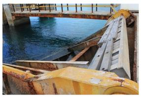
**Figure 5**. Major damage on movable bridge after Lua storm on March 2012.
