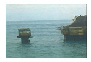
**Figure 3.** Significant damage of breakwater due to high wave on January 25<sup>th</sup>, 2012
