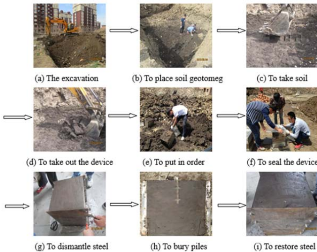
Figure 3: The process of taking soil and burying model piles
