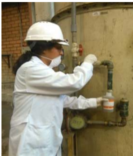
Figure 1: Sampling of gas scrubber.
