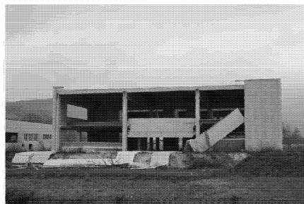
Figure 1. Collapses on precast concrete buildings and weakness of connections between primary and secondary elements.
