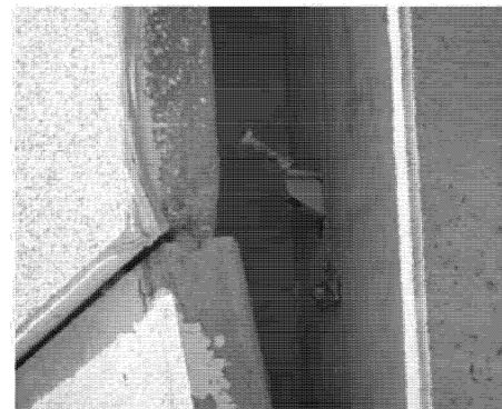
Figure 1. Collapses on precast concrete buildings and weakness of connections between primary and secondary elements.
