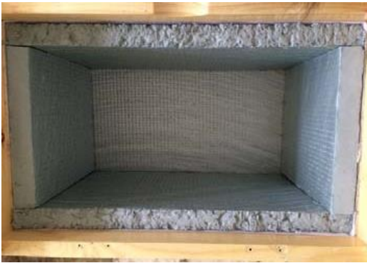
Figure 2: Interior wall of housing model
