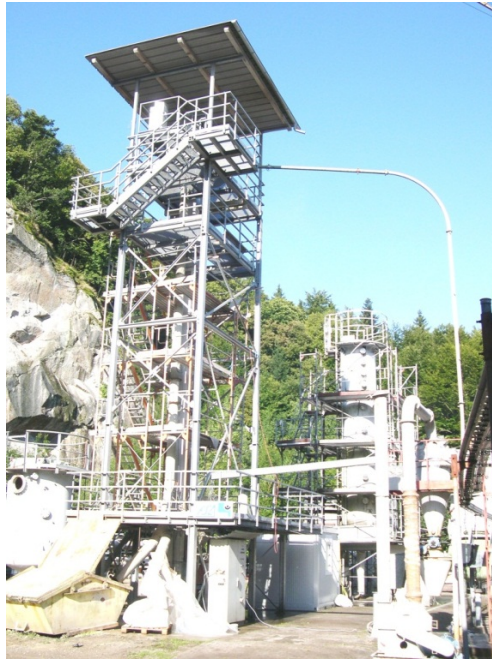
Figure 1: Double-leg bucket elevator used for the investigation
